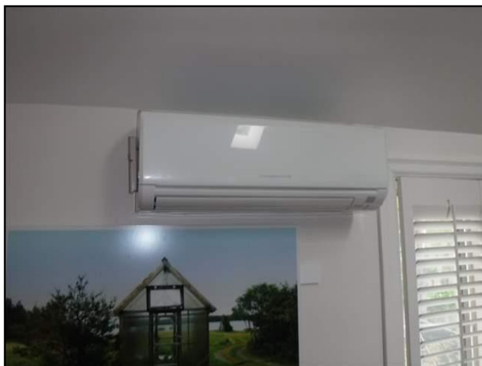
Ductless (Mini split) system
