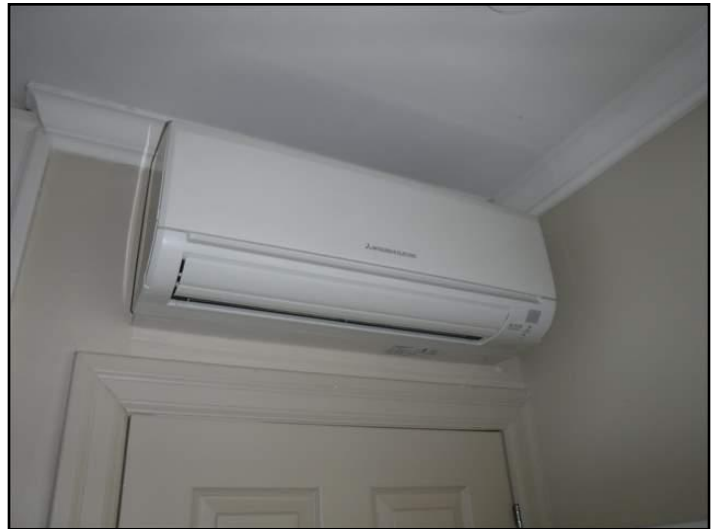
Ductless (Mini split) system
