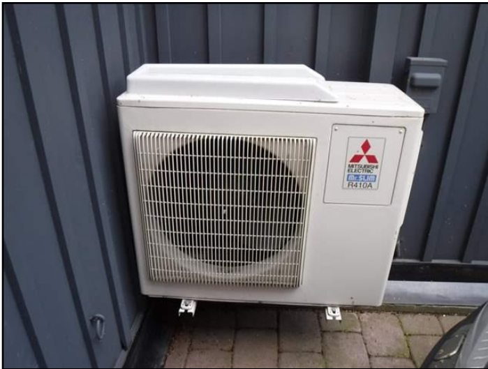
Ductless (Mini split) system
