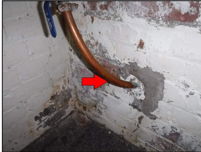
Upgraded water supply pipe
